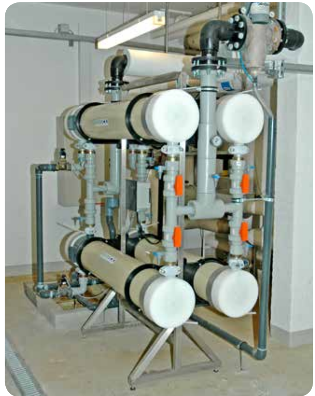
ENWA BIN-X complete ultrafiltration system.
