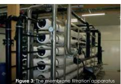
Figure 3: The membrane filtration apparatus (60 m3/h capacity) at Hardingsmolt AS. Built by Aquasulfat project partner ENWA.
